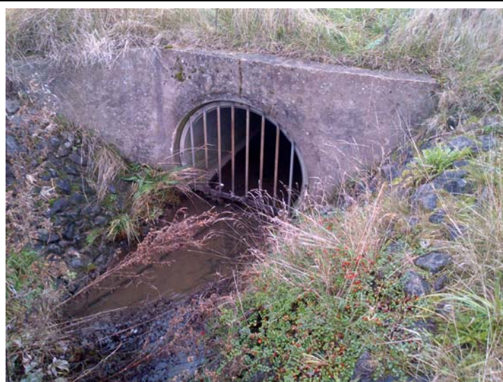
Figure 4-1: 1300mm diameter culvert entrance
